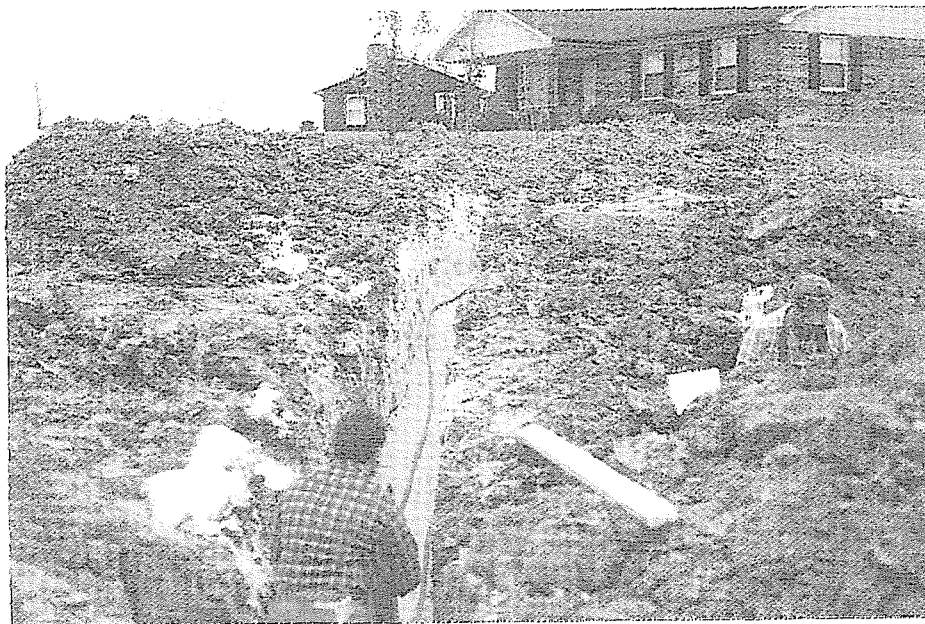
The geothermal heating and cooling system is more efficient because it uses the earth as its heat source.
